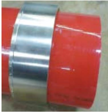
2. Push the sliding sleeve onto the pipe. Caution! The inner bevel must point towards the end of the pipe.
