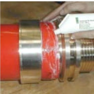
7. Cover the entire circumference of the pipe uniformly with lubricant in the area of the joint.
