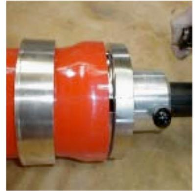
3. Expand the pipe twice with a 30° offset. The sliding sleeve must not be in the expansion zone. Minimum interval: 2 x the length of the sliding sleeve!
