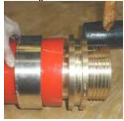
6. There must be a uniform gap between the fitting collar and the pipe end. If necessary, the position of the fitting must be aligned by means of a rubber hammer immediately after insertion. Caution! All the sealing ribs must be covered by the pipe!
